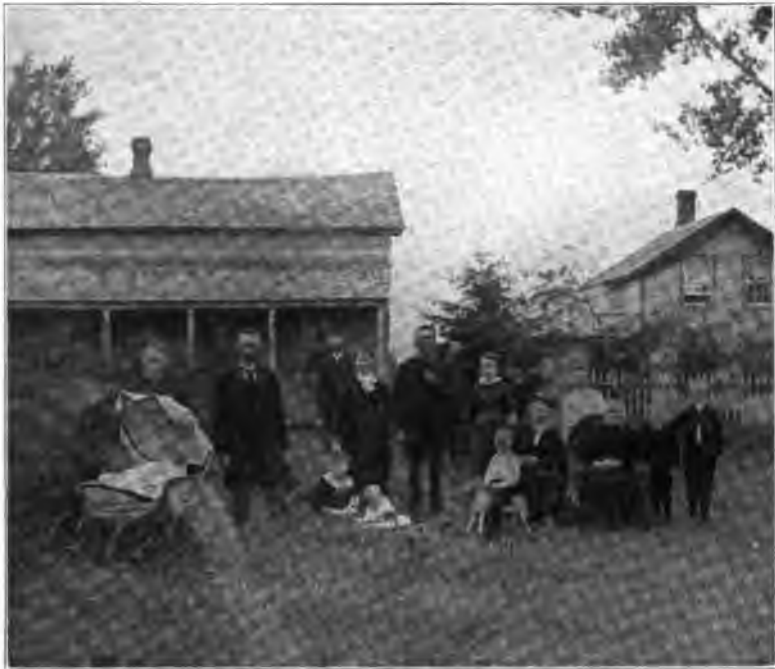
First Frame Dwelling in Howard Township, Story County, built by the Heglands in 1857. This house was the first meeting place of the Lutherans in this township
